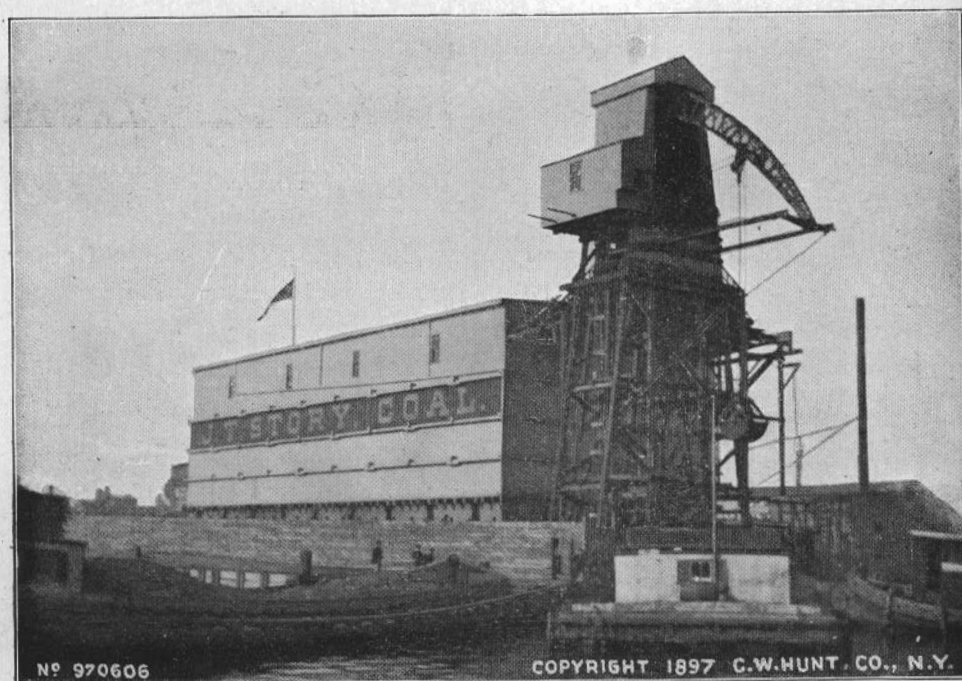
J. T. Story, Coal Yard, Brooklyn, N. Y. The pocket holds 7,000 tons of coal. The coal is hoisted with a two-ton Hunt Steam Shovel, and distributed in the building by two automatic cars on independent tracks.
