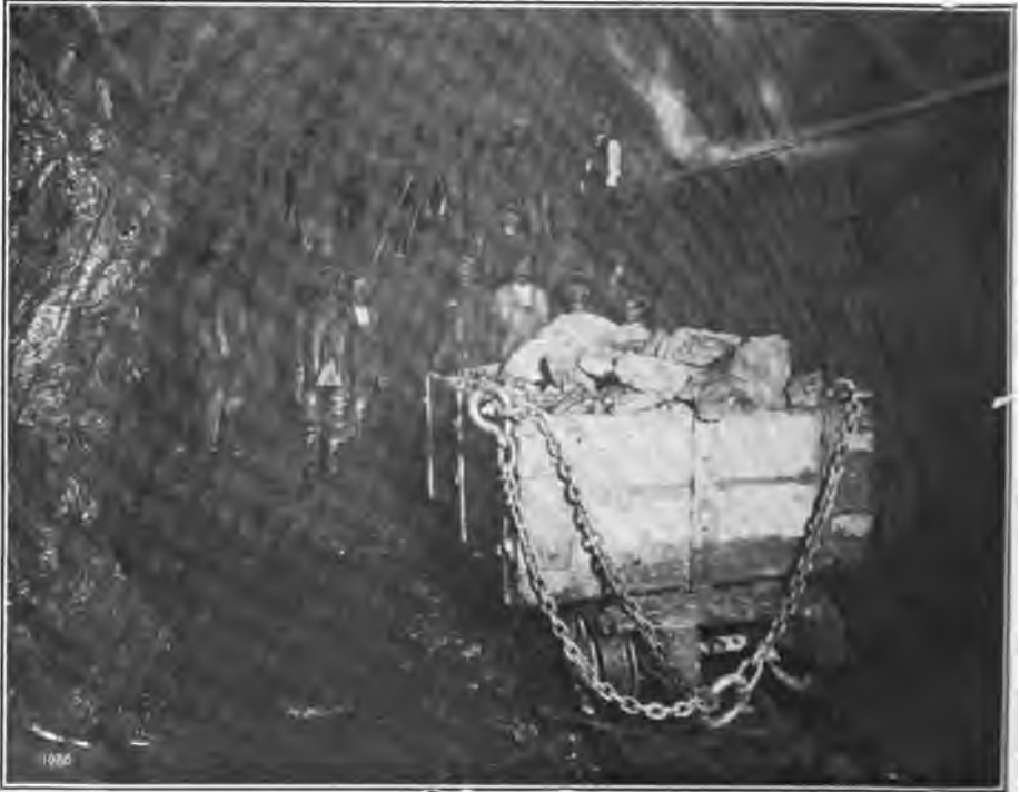
EXCAVATING IN THE HEADING ON THE NEW YORK SIDE.
