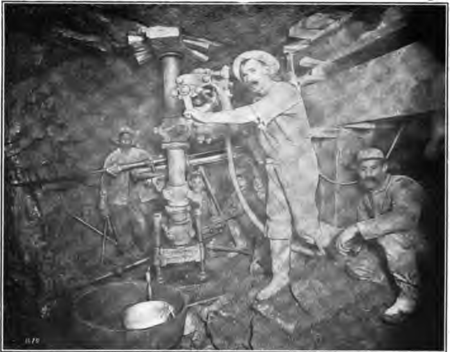
ROCK DRILL IN THE HEADING UNDER EAST RIVER.
