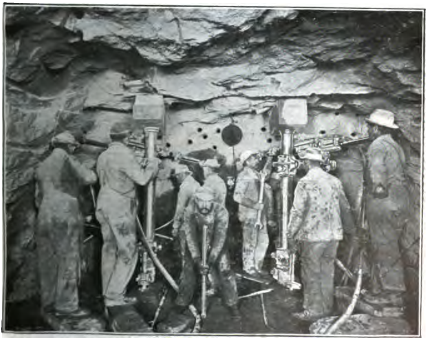
AIR DRILLS DRIVING A HEADING.
