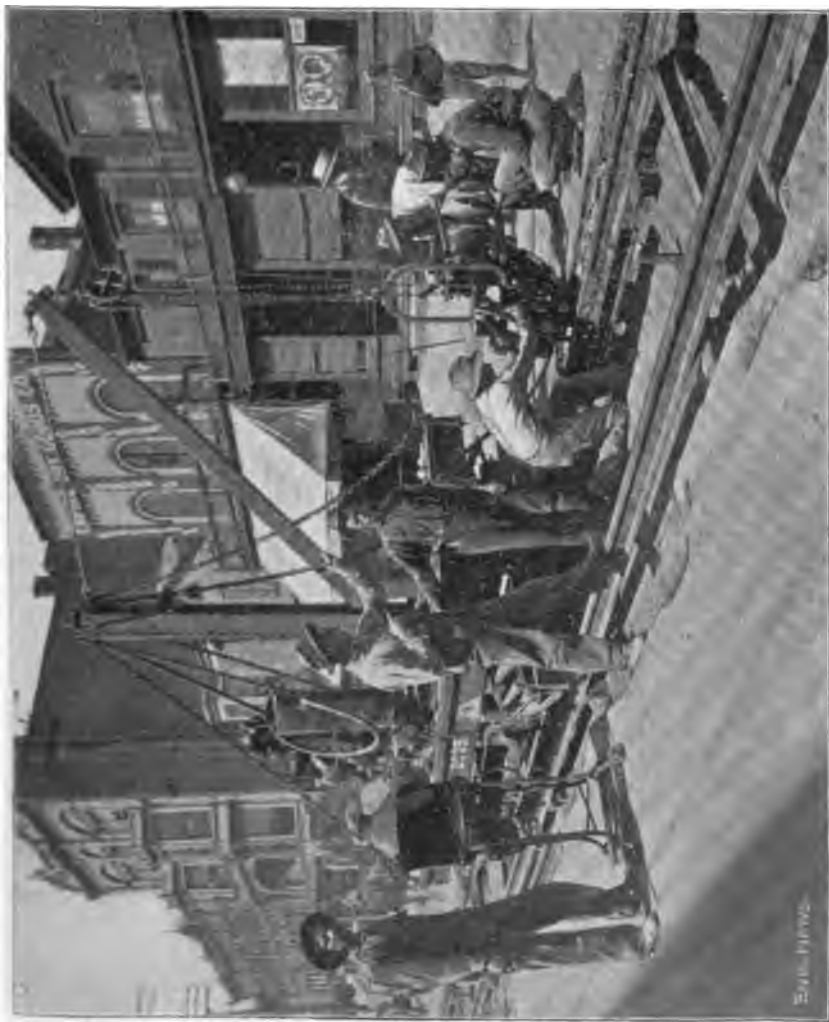
RIVETING PLANT FOR RAIL JOINTS, SCRANTON RAILWAY CO. (Showing reinforcing rail under the joint, and also one of the steel cross ties at the right.)
