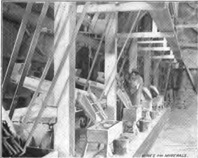
CONCENTRATION FLOOR, MODOC MILL, SHOWING BATTERY OF HOOPER PNEUMATIC CONCENTRATORS.
