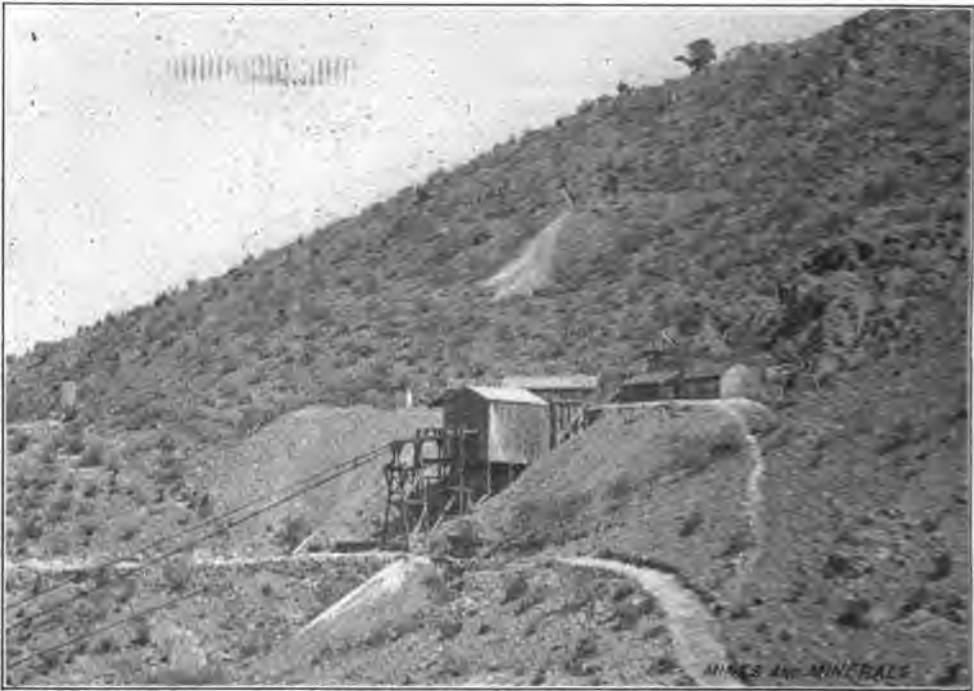
MODOC MINE, SHOWING UPPER TERMINAL OF TRAMWAY.
