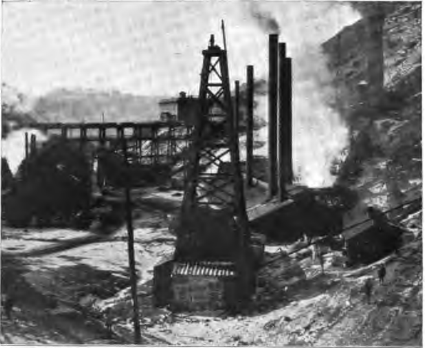
AIR-LIFT WELL OF CAMBRIA MINING COMPANY, WYOMING.
