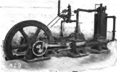
Class "G" Compound Air Compressor.
