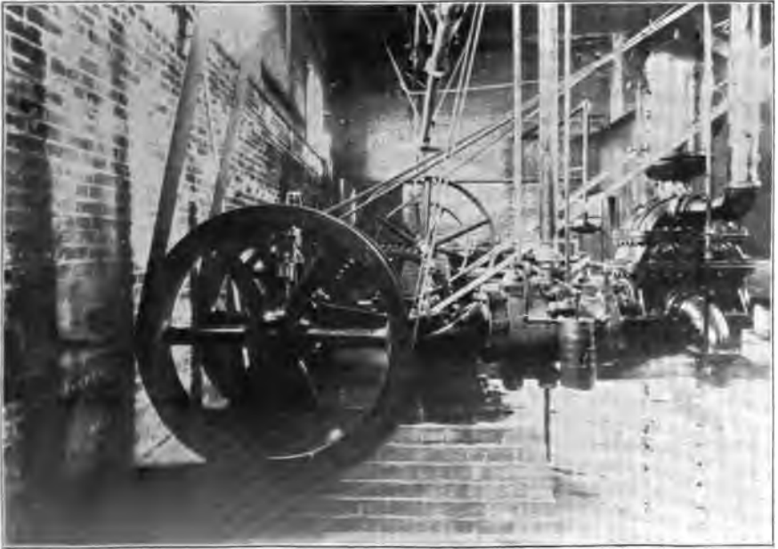
FIG. 6—AIR COMPRESSOR PLANT, MOON ISLAND SEWAGE RESERVOIR.
