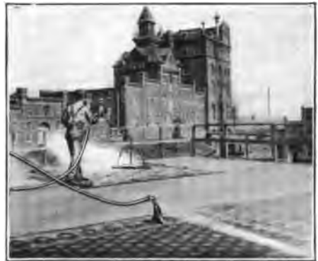
FIG. 1—CARPET BEING CLEANED OUT IN THE OPEN AIR.
