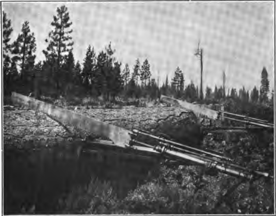
THE PNEUMATIC SAW AT WORK.
