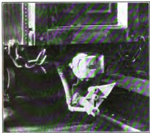
END VIEW, TRETHEWEY STEAM AND AIR COUPLING.
