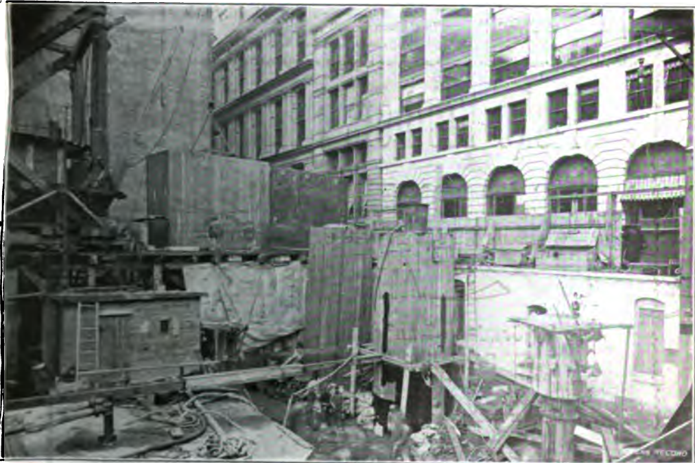
SINKING CAISSONS FOR PIER FOUNDATIONS, HANOVER BANK BUILDING.
