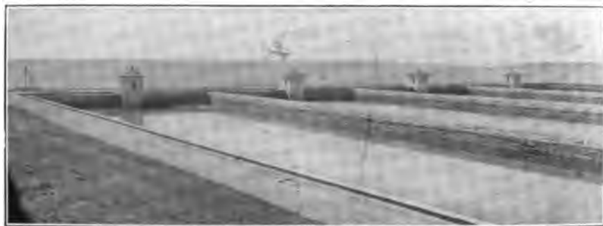
FIG. 1—MOON ISLAND SEWAGE RESERVOIR, BOSTON, MASS.
