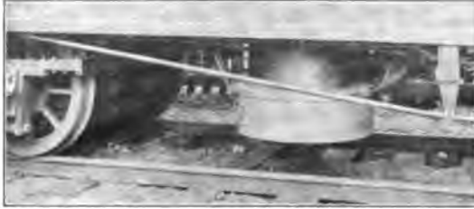
FIG. 2—TURRET CONTROLLER MOUNTED UNDER CAR.
