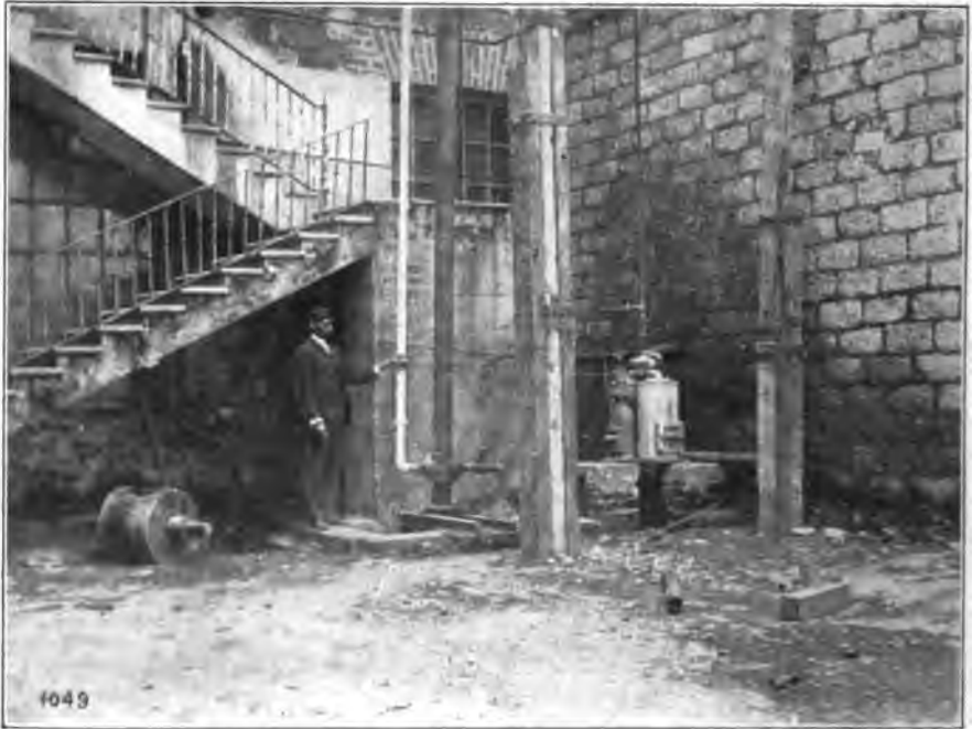
FIG. 1.—SHOWING PIPING AT WELL NO. 1, THE MACHINE TO THE RIGHT BEING THE DISCARDED PULSOMETER.
