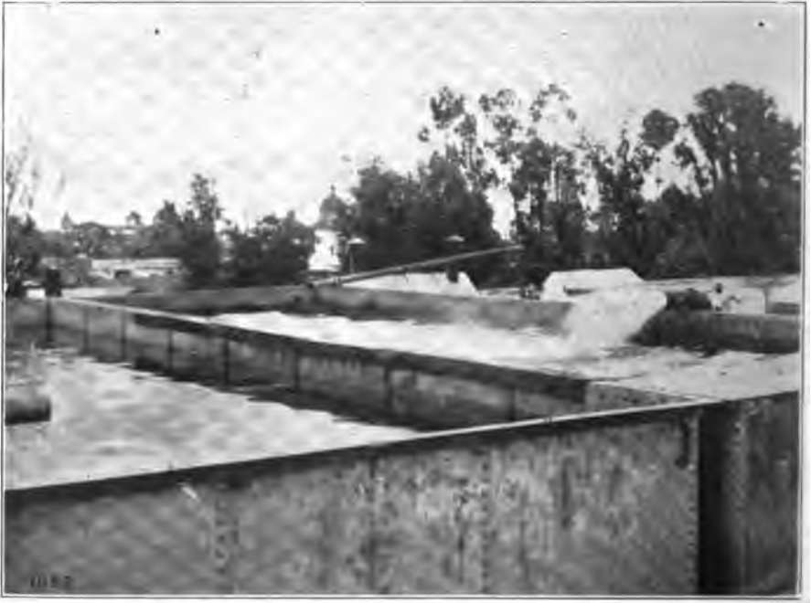
FIG. 3—SHOWING 5-INCH DISCHARGE OF WATER INTO THE TANKS ON THE ROOF.
