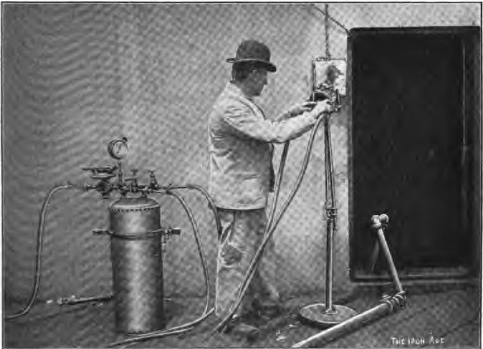
THE TYNAN ANNEALER WORKING ON ARMOR.
