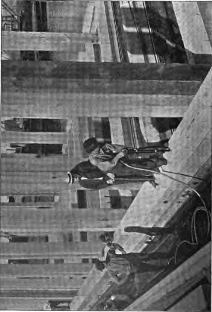
PNEUMATIC RIVETING HAMMER FOR CRIB-WORK.
