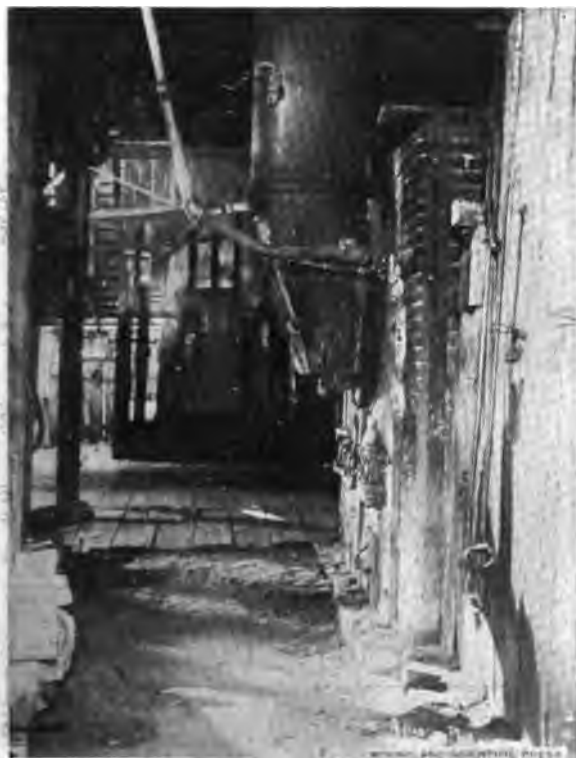
AIR PIPE FROM COMPRESSOR ENTERING BOILER, SPRING HILL MINE.
