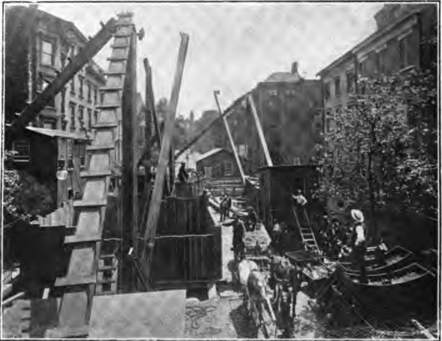
ENTRANCE TO THE SHAFT IN JORALEMON STREET, BROOKLYN.
