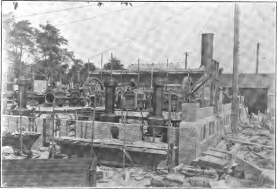
PARTIALLY COMPLETED POWER PLANT OF THE CLEVELAND STONE COMPANY.
