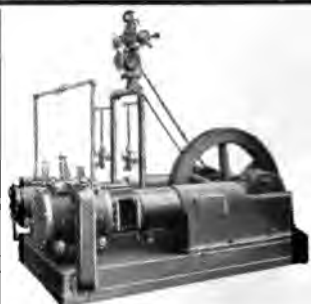
Class F. Steam-driven Two-stage Air Compressor.
