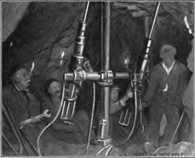
WATER-LEYNER AIR DRILLS MOUNTED ON COLUMN WORKING IN STOPE, AT MODOC MINE.
