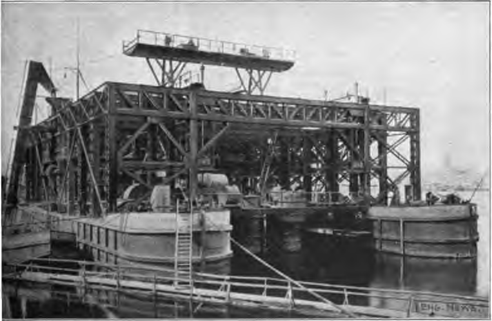
FIG. 3—VIEW OF MAIN CAISSON IN OPERATION.
