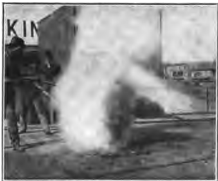
FIG. 3—CLEANING WITH OPEN NOZZLEMAN.
