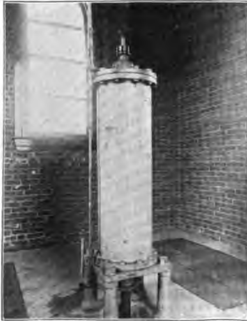
FIG. 2—PNEUMATIC CYLINDER FOR LIFTING FLUSH GATE.
