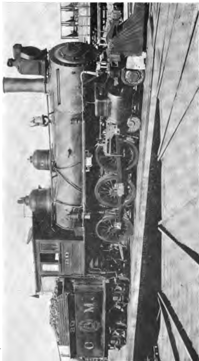
LOCOMOTIVE FITTED WITH PRIEST SNOW FLANGER.
