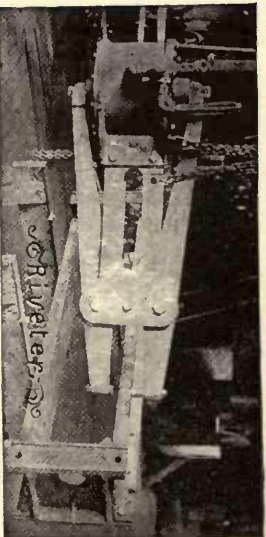
STAY BOLT CUTTER AND RIVETER IN USE IN RAILROAD SHOPS.
